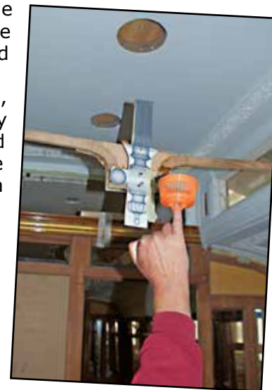
Air admission cage printed and trialled in-situ.
