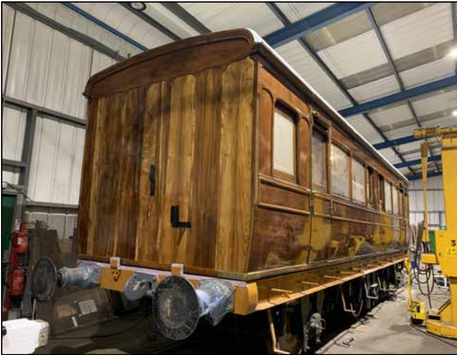
The end panels shown here on June 10 on GER No. 8 were made up from teak supplied by the LNERCA. Andrew Daniel machined up and joined narrower sections of teak to fabricate wide panels that have now been fitted and varnished. Photo: Dave Cullingworth.
